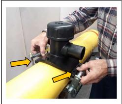
1. After the pipe has been scraped, hook both ends of the clamping device into the holes on the lip of the tapping tee.
