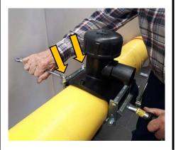
3. Alternately tighten each bolt on the side opposite the handle (see steps 4 and 5).
